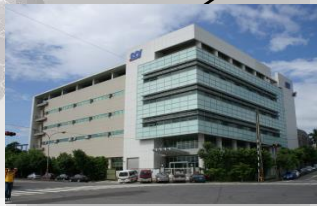
Nantou, Taiwan SDI Plant , TBT , CSM
